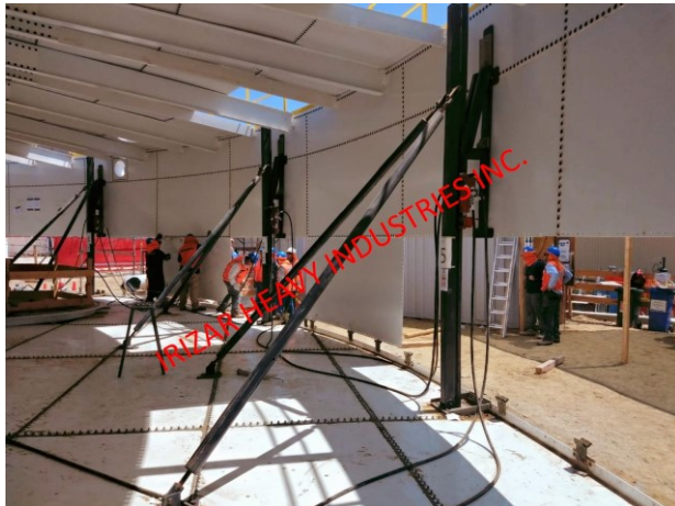
Bolted Tanks Lifting Jacks
