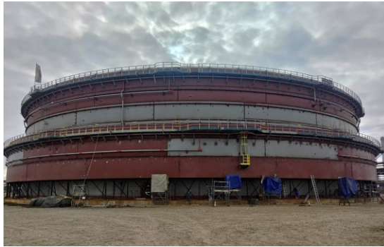
Double Wall Tank Lifting
