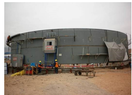
AGW-1 (Compatible with Lifting Jacks) Circumferential Welding for Outside the Tank
