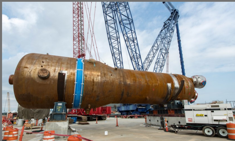
July 2017. Irizar Welding Rotator Model WR 1200 MT At Nuclear Construction Site in Georgia Power Plant Vogtle, USA Westinghouse Nuclear Power Generator AP 1000 PWR
