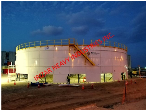
Bolted Tanks Lifting Jacks
