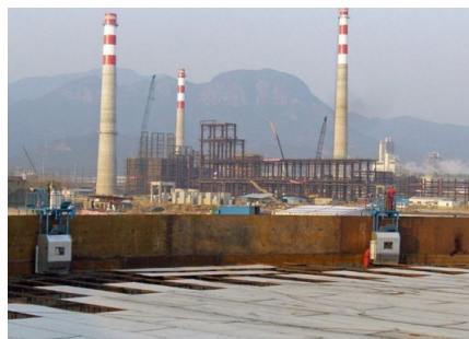
AGW-2 (Traditional Method) Circumferential Seam Inside/Outside simultaneously
