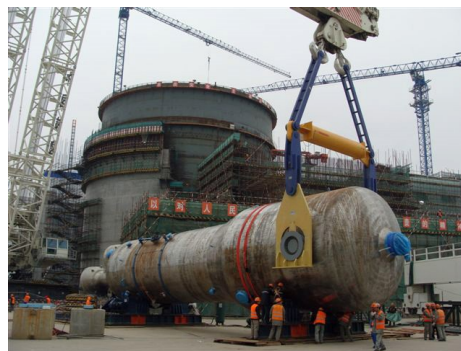
March 2013. Irizar Welding Rotator Model WR 1200 MT Nuclear Power Generator at Haiyang, Shandong, China Westinghouse AP 1000 PWR
