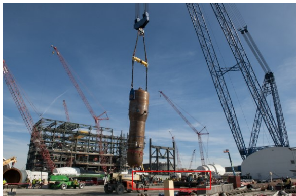
January 2017. Irizar Welding Rotator Model WR 1200 MT Nuclear Power Generator at VC Summer, South Carolina USA Westinghouse AP 1000 PWR
