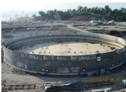
AGW-1 (Traditional Method) Circumferential Welding for Outside the Tank
